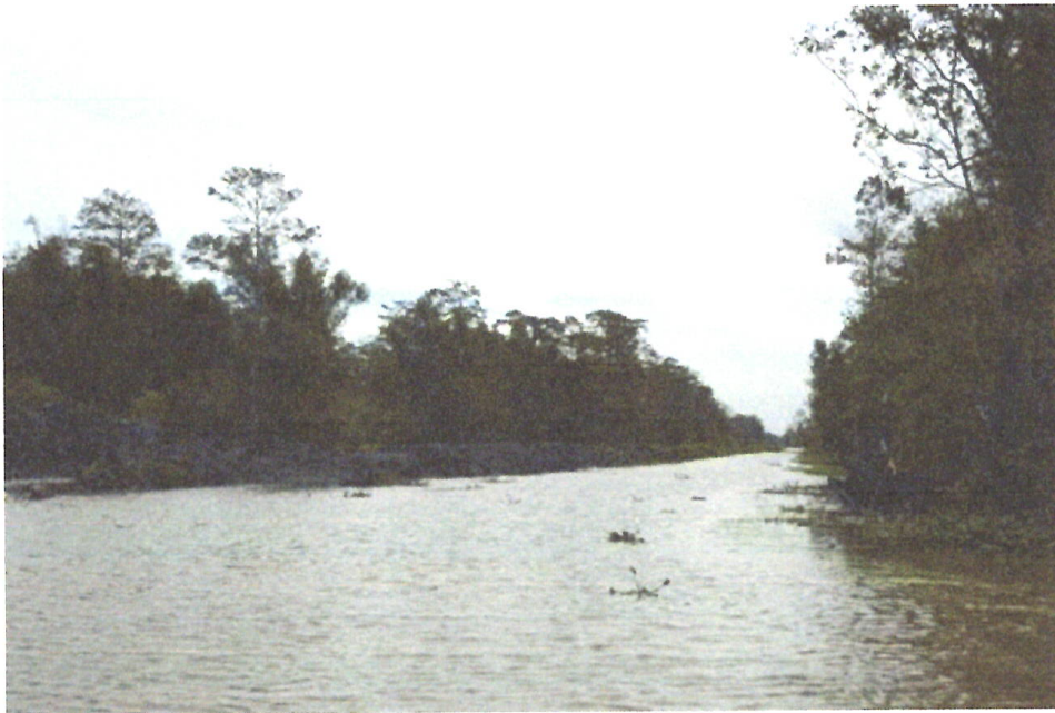
Unnamed bayou dam
