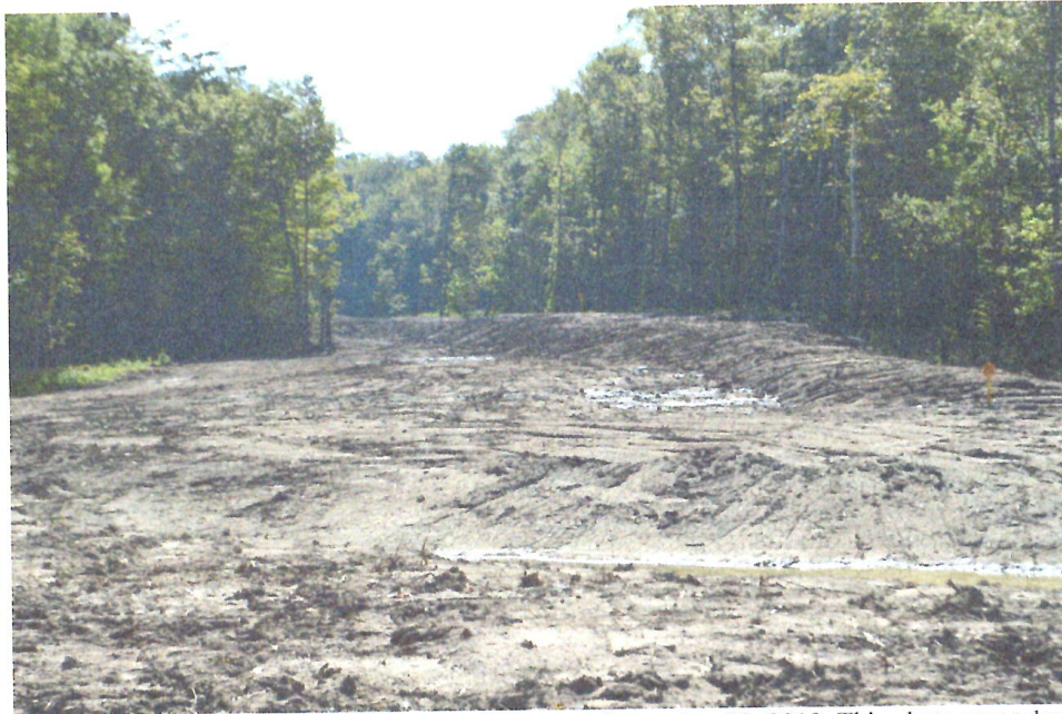
Figure G: This Photo was taken by Dean Wilson on September 20, 2018. This photo was taken facing southeast along the pipeline right-of-way at approximately 30.11311944, -91.54972222. This photo depicts an existing spoil pile on the south side of the pipeline right-of-way, and pipeline markers on top of the spoil pile.
