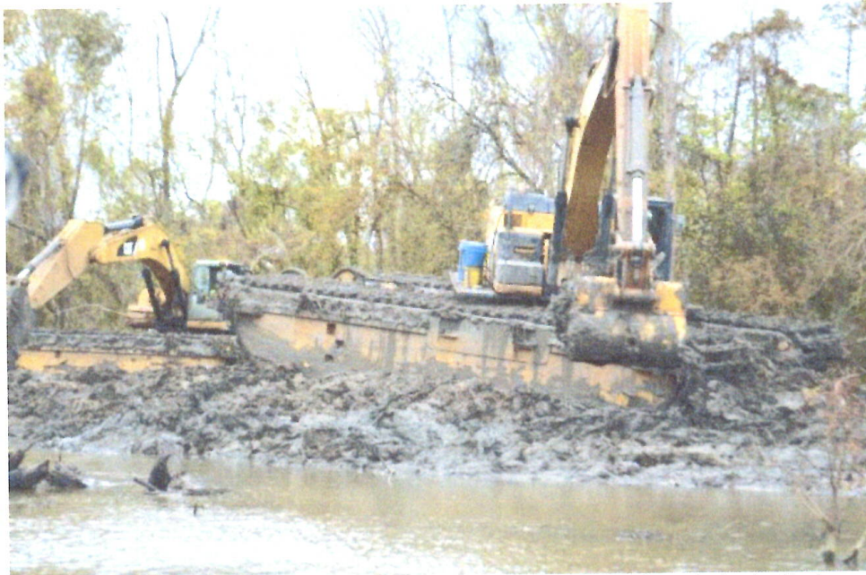
Figure A: This photo was taken by Dean Wilson during the monitoring trip in the Basin on December 7, 2018. This photo was taken approximately 1.5 miles east of Flat Lake Pass. Approximate coordinates 30.08572778, -91.41138889. Figures A-C depict active construction in the area and a lack of erosion or sediment control measures in place.
