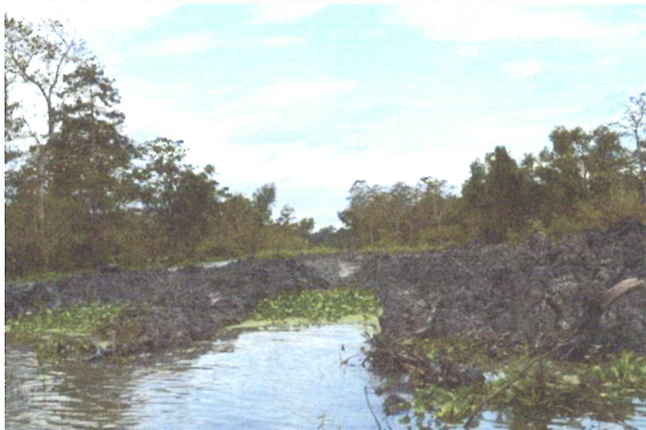
Spoil bank, no gaps
